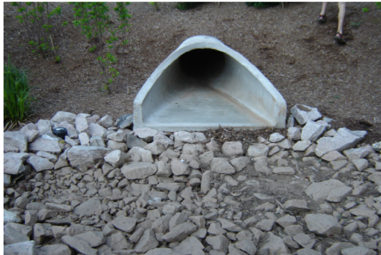
Figure 25: Properly utilized forebay (NCDENR 2007)
