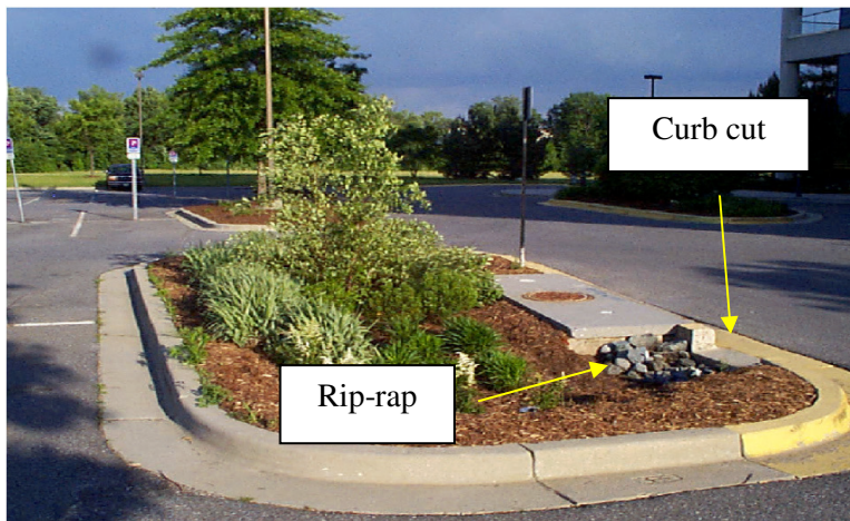
Figure 26: Curb cut inlet system (NCDENR 2007)
