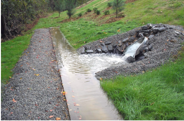
Figure 12: Improper entry to level spreader (Winston et al. 2010)
