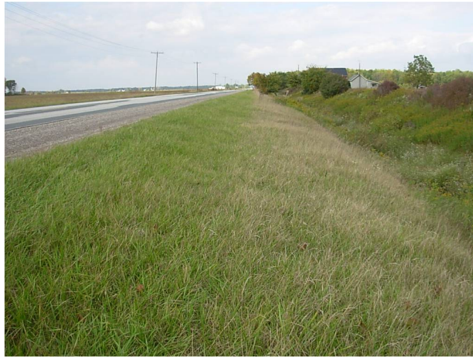
Figure 3: Roadside vegetated filter strip (TWG 2008)
