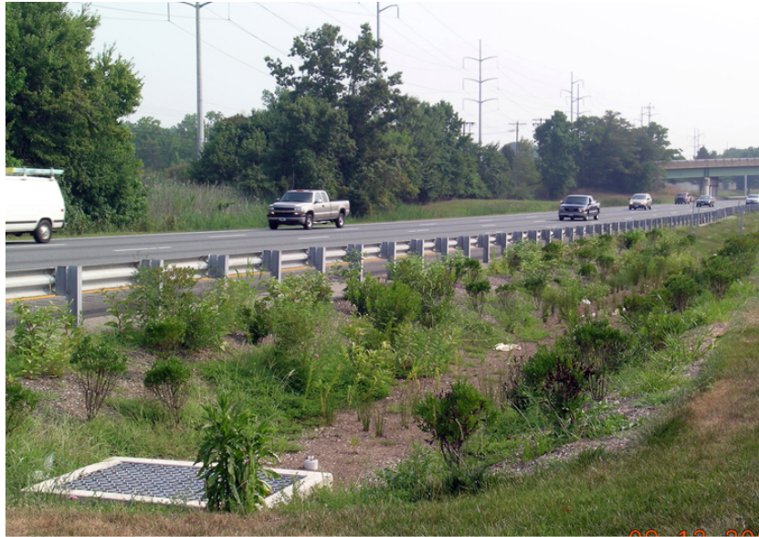
Figure 5 Highway median bioretention in Delaware (DelDOT 2012)
