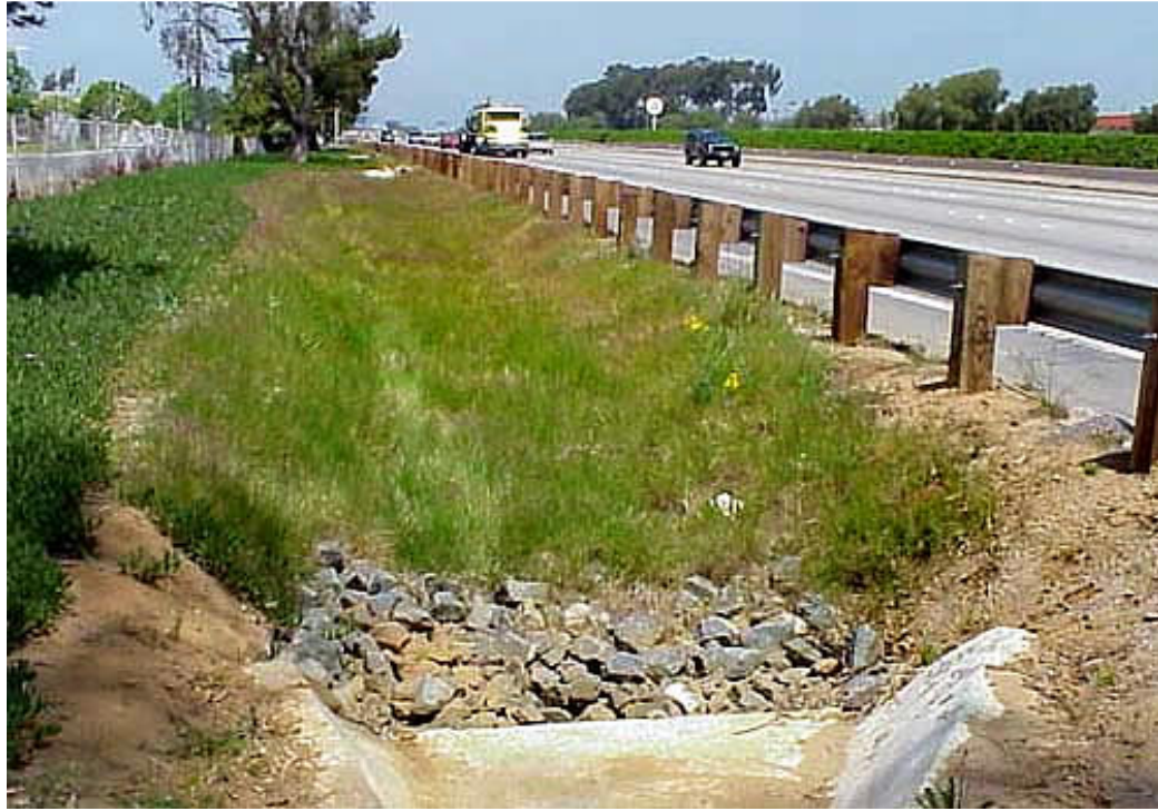
Figure 4: Roadside Swale (CalTrans 2012)
